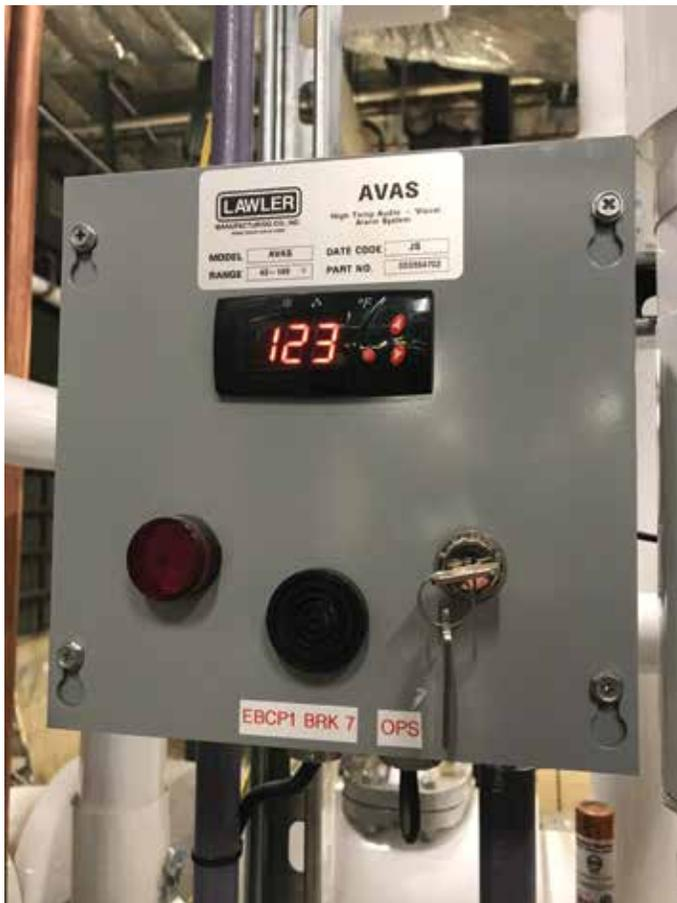
Designers should note that some regulations require specific safety controls on DHW systems. These controls must provide a fail safe shut off of the hot water supply to the central mixing valve if the temperature leaving that valve exceeds the valve's setpoint by a specific value, such as 10 °F. The system must also provide a visual and audible alarm, and only allow a manual reset of a detected fault condition. Figure 3-11 shows an example of such a controller.
